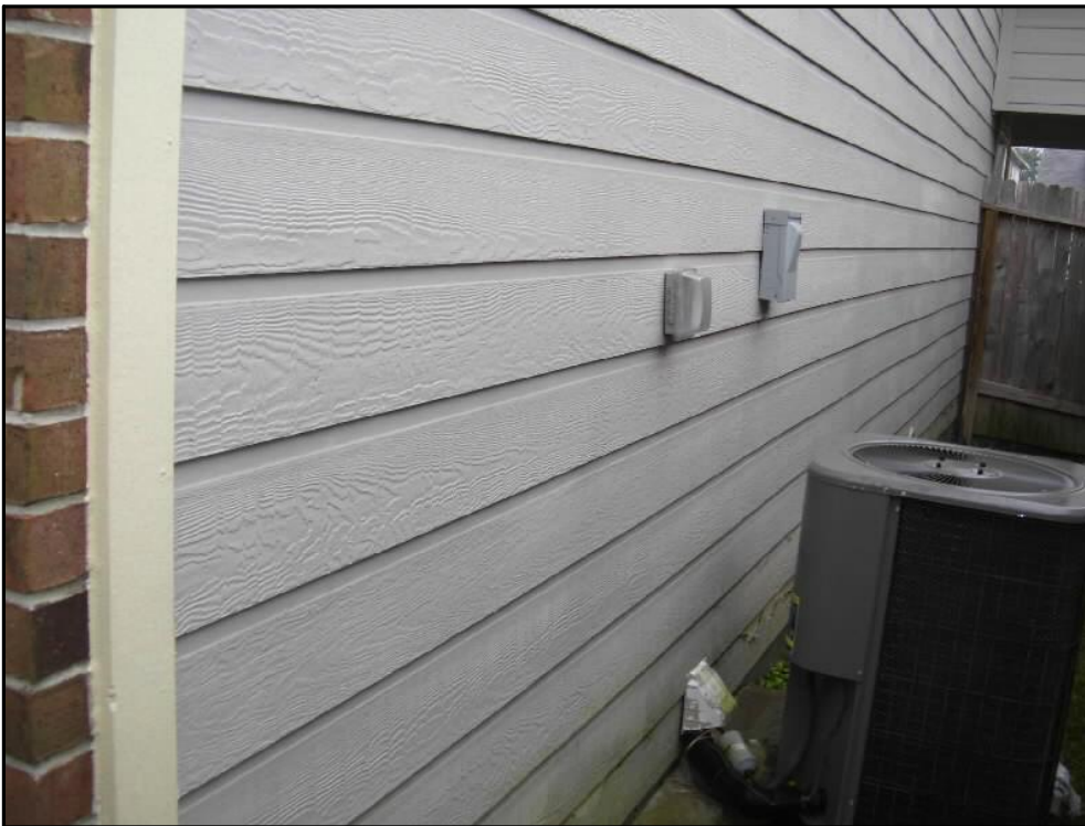
2410 CHUCKBERRY ST GENERAL VIEW 2
