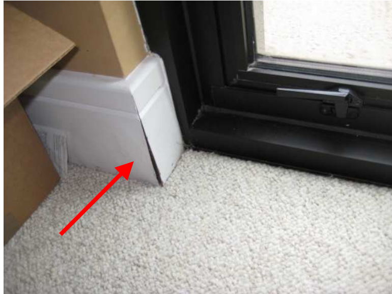
Possible water stains observed on lower corner of garage wall near door; moisture meter indicated area was dry at time of inspection.
