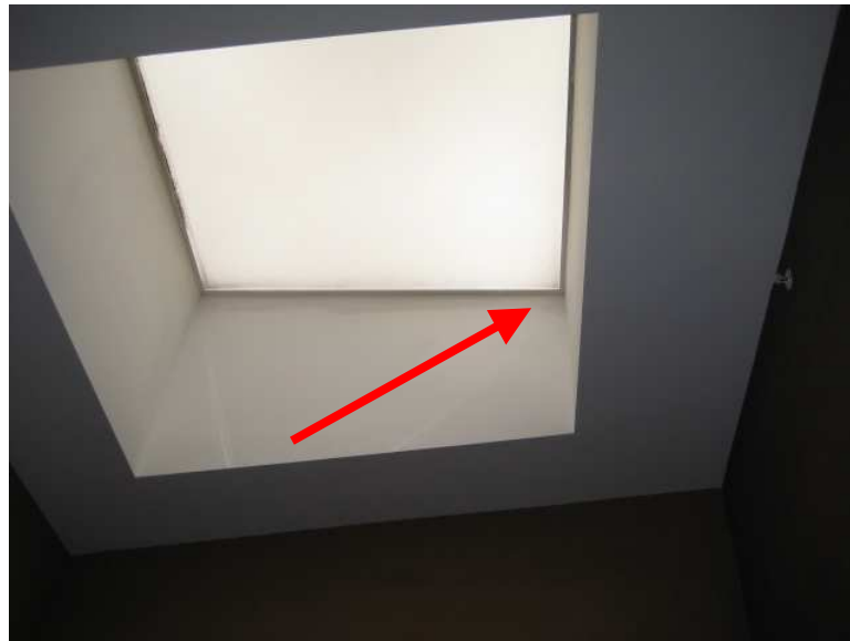
Water stains around skylight over stairway/kitchen area.
