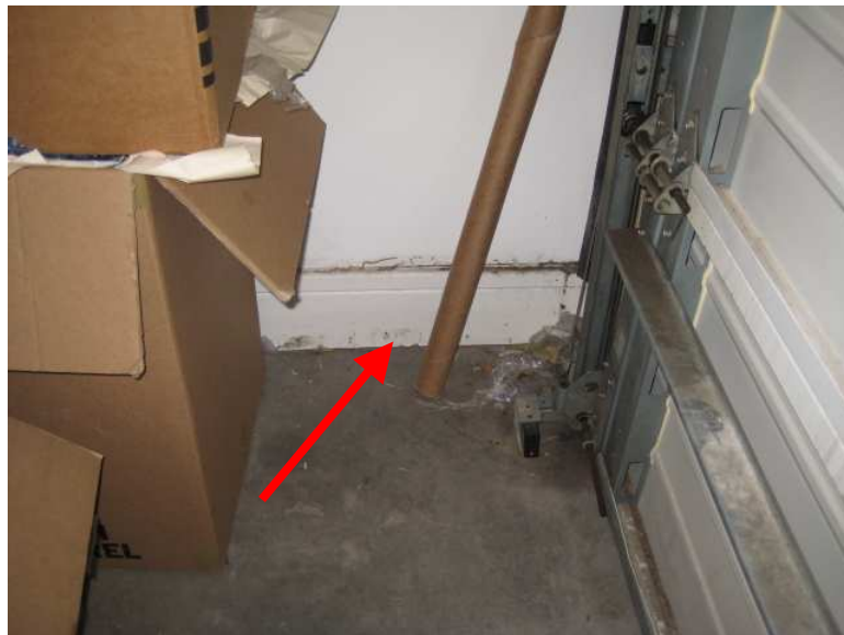
Possible water stains observed on lower corner of garage wall near door; moisture meter indicated area was dry at time of inspection.
